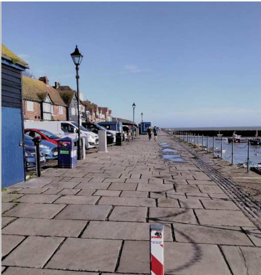
Figure 2 – Photo of site
